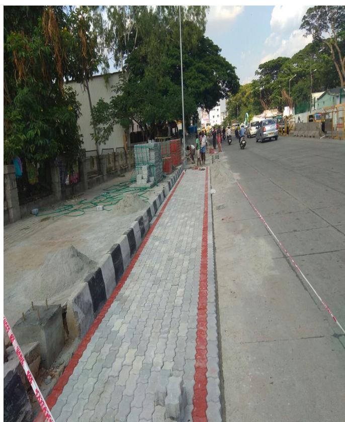
Bufferzone and Footpath Paver block laying Work in Progress
