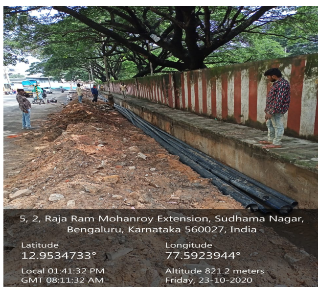
HDPE Pipe line laying work in Progress.
