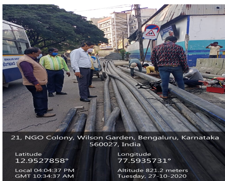
HDPE Pipe line laying work in Progress.
