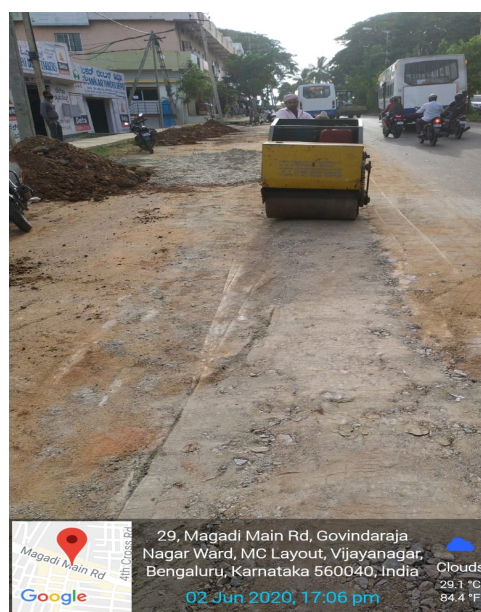
BWSSB Water Supply line trench Restoration work.
