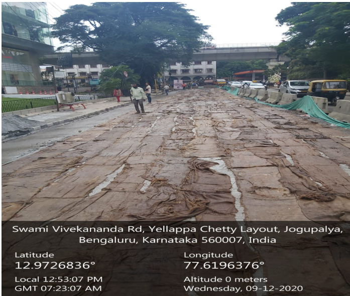
White Topping work in Progress
