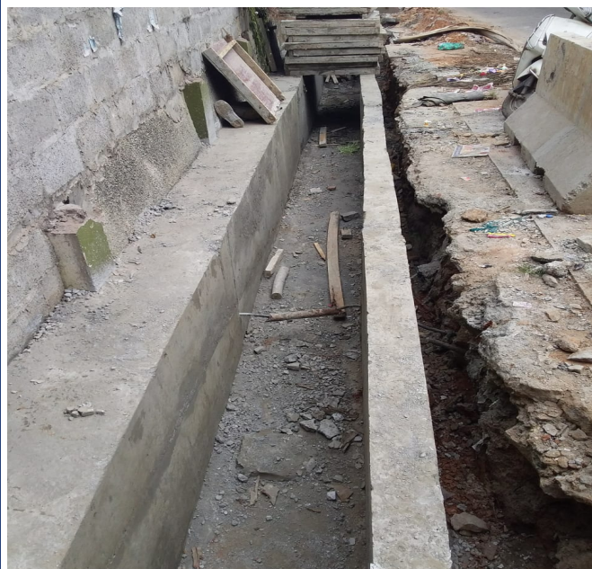
Drain work and Access Chamber Construction work in Progress.
