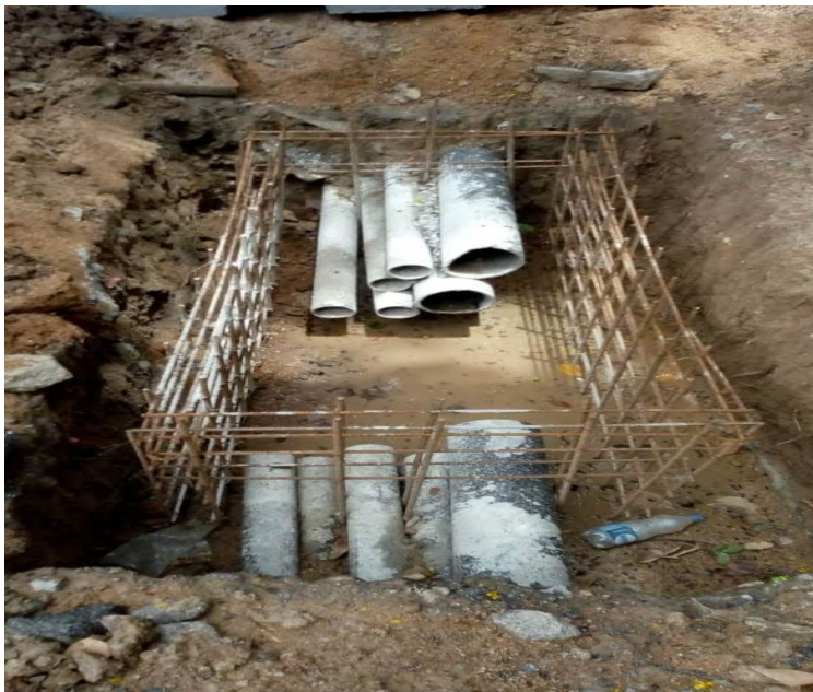
Drain work and Access Chamber Construction work in Progress.
