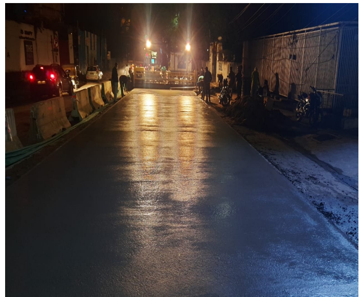
White Topping work in Progress
